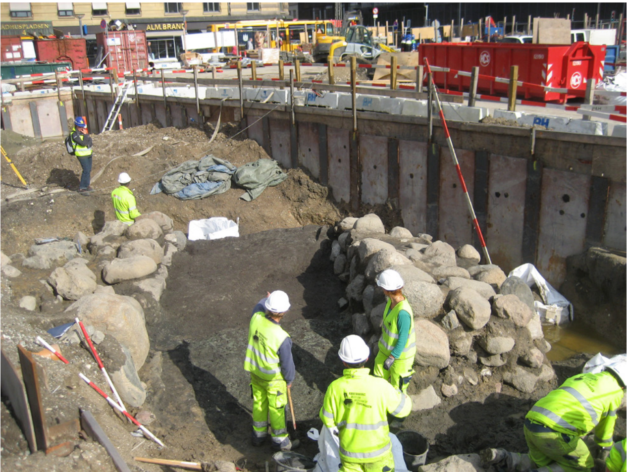
Fig. 2: New knowledge and prioritizing! ... Key words in the management of developer payed archaeology and characterising, for instance, Museum of Copenhagen's very large excavation in the city centre prior to the construction of a new metro line
