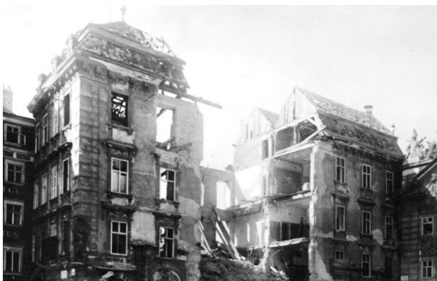
Figure 6: The badly damaged building Am Hof on 19 July 1946 (BDA Photo archive)
